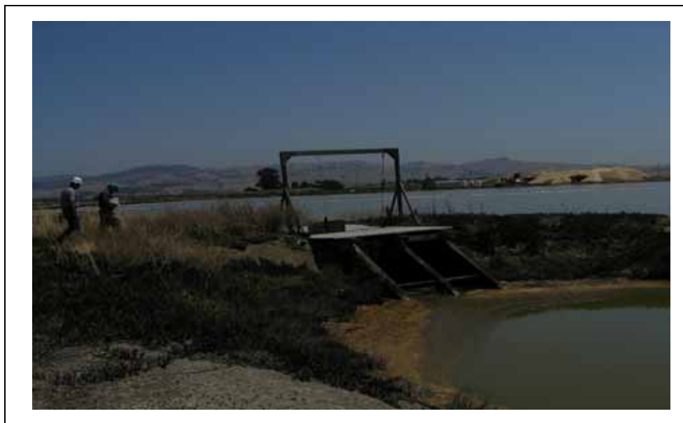
Photograph 10: Example of a brine gate. Camera facing northeast.
